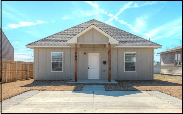
Photo is of a similar home by the builder.
